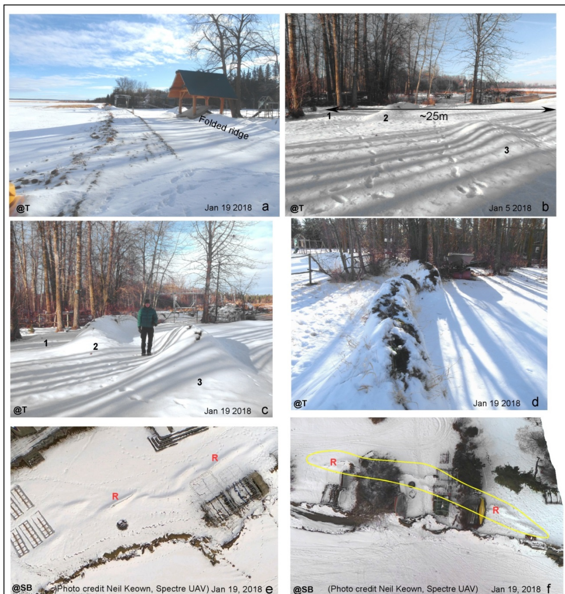
789 790 Figure 6. Inland ground deformations. (a) View of undeformed lake ice in contact with shore, 791 and folded, deformed ground onshore beneath the gazebo structure at the Thibeault site, Lac. Ste. 792 Anne, January 19 2018. (b) Multiple inland ground folds (numbered) at the Thibeault site, Lac. 793 Ste. Anne, January 5 2018. Photo (b) taken 5 days after the icequake, during which time folds 794 grew to about 0.5 m in height. (c & d) Photos taken two weeks later, during which time folds 795 have doubled in height and ruptured. (e & f) Aerial view (UAV imagery) of folded ground at 796 two sites near Seba Beach, Wabamun Lake. Ridges in photo (e) are about 0.3-0.4 m high and 7- 797 13 m long. Ruptures (R) are evident in some of the folds. (f) Ridges in photo (highlighted in 798 yellow) are about 0.4-0.5 m high and 5-8 m long. Locations of pictures are annotated in the 799 bottom left of the panels based on acronyms in Figure 1.
