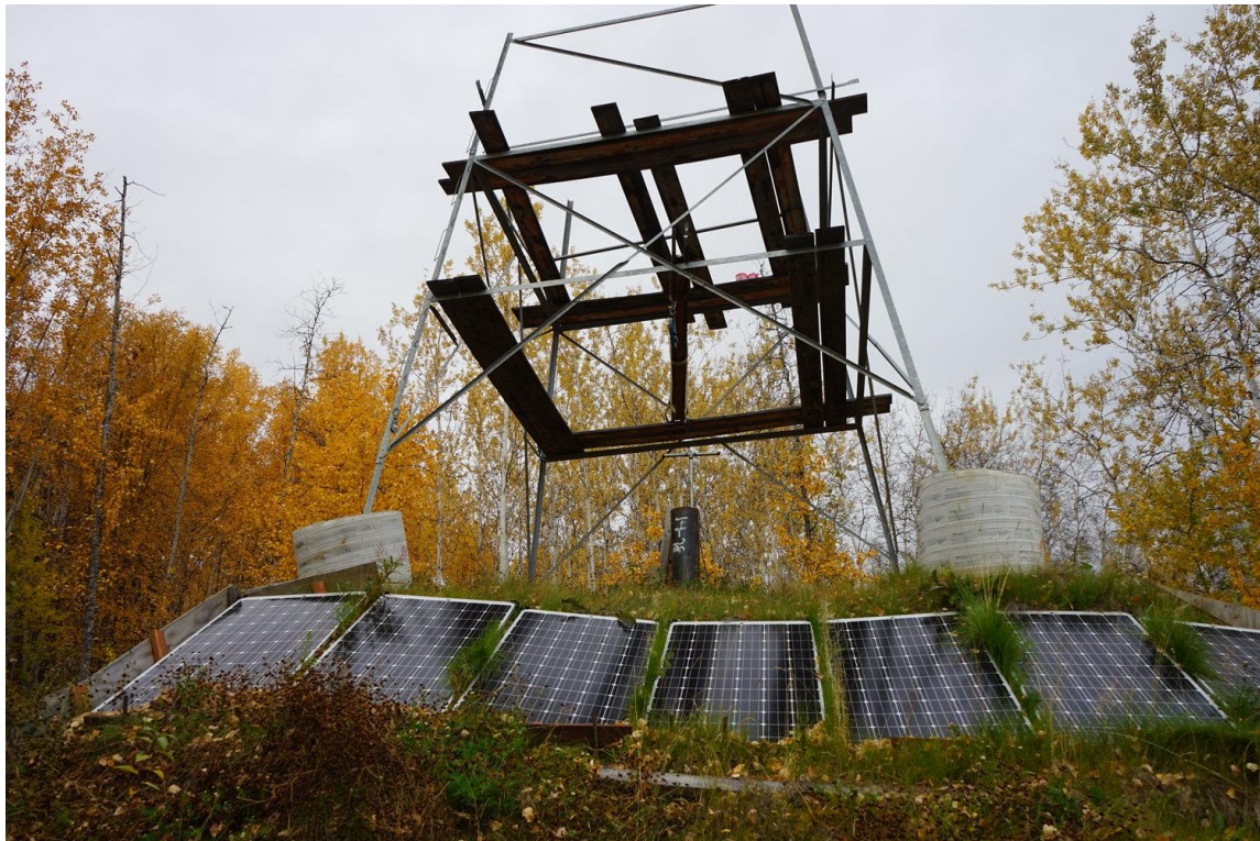
Figure A.13. Geothermal well used for heating the greenhouses. Solar panels power the down-hole pump.
