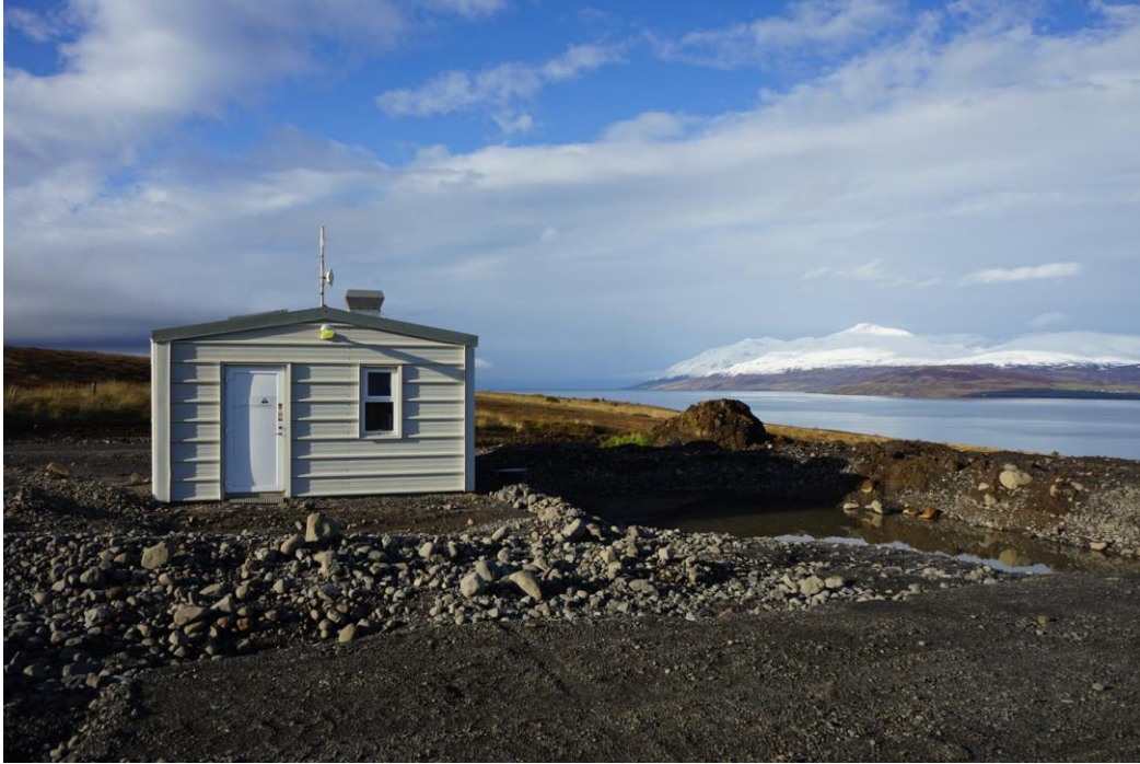
Figure A.25. One of two wellheads at the highly successful Hjalteyri field on the east shore of Eyjafjörður. Hot water is carried via buried pipeline to heat buildings in Akureyri, ~20km south. Such a small spatial footprint!
