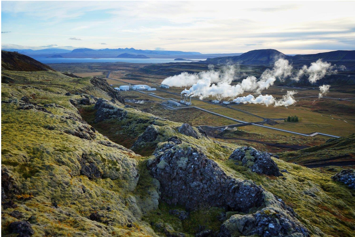
Figure A.20. Nesjavellir Power Plant, situated on the northern flank of Hengill Volcano.
