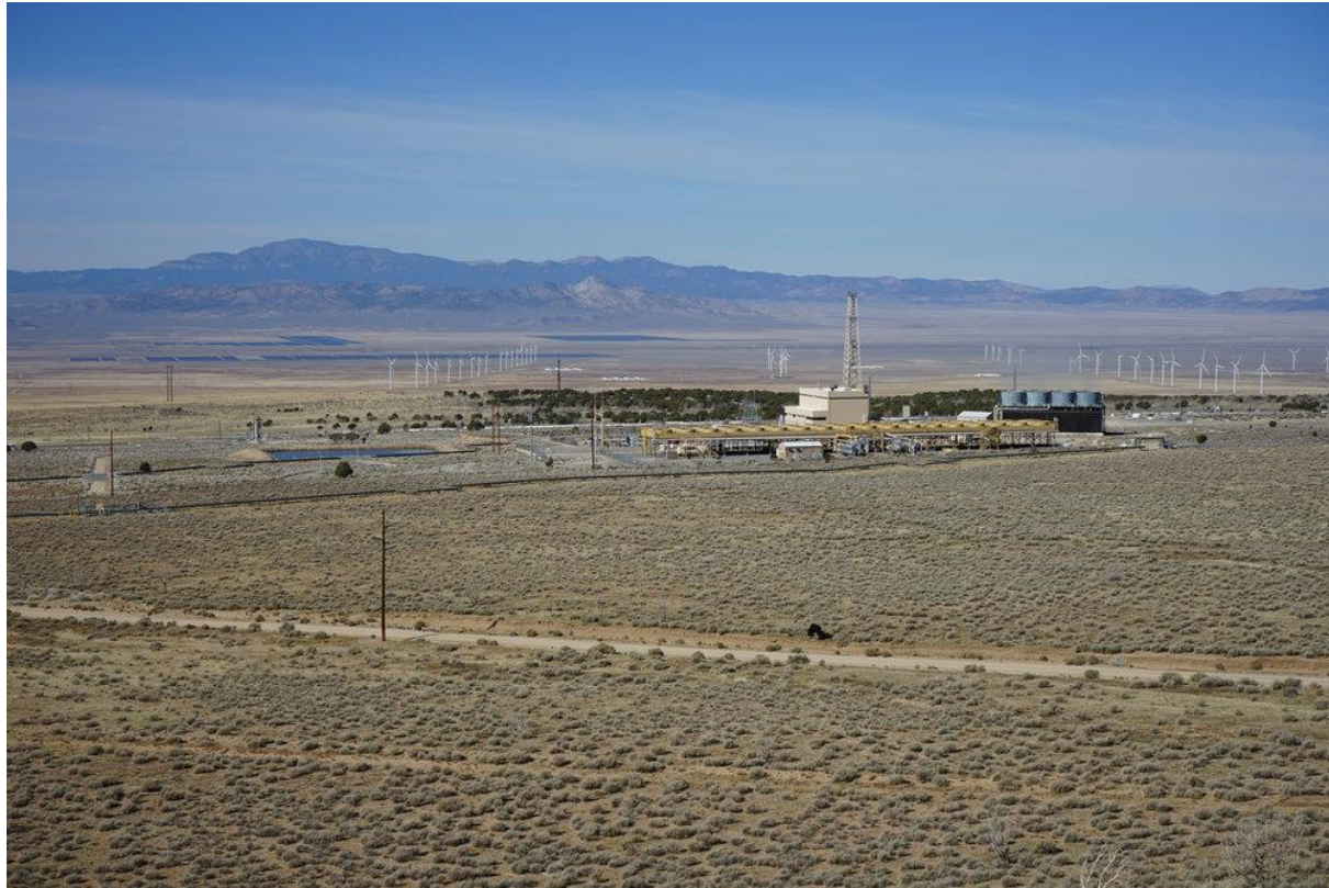
Figure A.38. The Milford Renewable Energy Corridor, looking WNW. In the foreground, the Blundell Geothermal Power Plant produces 34 MW of power from a hydrothermal system that appears to be bounded by a steep fault that roughly corresponds to the treed hillside behind the plant. The Milford FORGE site will be between the rows of wind turbines on the right side of the image. Across the valley, a large solar farm also produces electricity.
