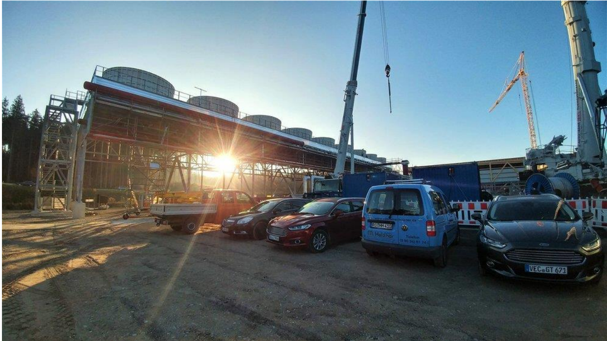
Figure A.48. Cooling towers at Holzkirchen. Working fluid must be cooled to create a pressure differential to drive the turbines.
