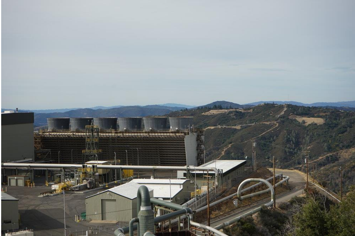
Figure A.41. One of the many power plants at the Geysers geothermal field, the world's largest geothermal power producer. In the background, numerous steam pipes from various wells are visible.
