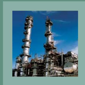
Sarnia's new gasoline hydrotreater had a flawless start-up December 2002.
