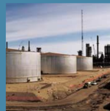
Tank farm at the new Scotford Upgrader.
