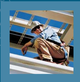
Lonnie Erickson, a welder with one of Shell Canada's contract companies, measures steel at the Waterton Complex.
