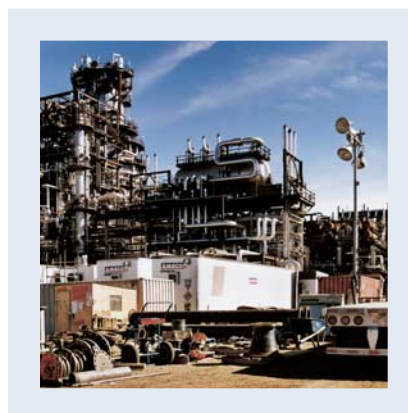
The atmospheric and vacuum units at the new Scotford Upgrader.
