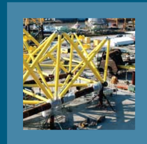
Platform under construction for the SOEP Alma field.
