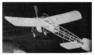
The cross-Channel monoplane was of all wood construction, covered with cloth. The wing warping system, instead of the modern aileron, was used to bank the plane. The three cylinder, 26 h.p. motor which pulled No. 11 across the channel in 37 minutes was especially built for Bleriot by Anzani.
