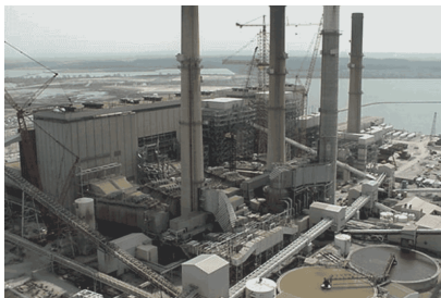
A coal plant being retrofit with capital intensive ($200M) pollution abatement equipment.
