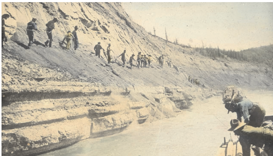
View of workers directly mining oil sand along the Athabasca River, although the source of the lantern slide is unknown, the material obtained was likely for use in paving roads in Edmonton in 1915. The oil sand lies immediately above the hard carbonate shelf. This image is freely available from Library and Archives Canada.
