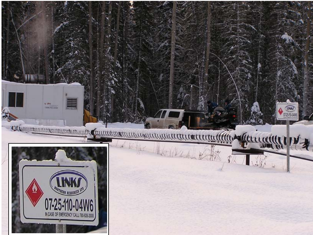
Figure 6.16: Photograph of producing Quaternary gas well 07-25-110-04W-6. Well number is clearly visible in the photograph. Compressor is attached with the well in order to pump gas in the gathering pipe lines. Compressor is seen the top left of the figure. This well is 700 metre south of the seismic and ERT line. Photograph taken by the author in January 2005.
