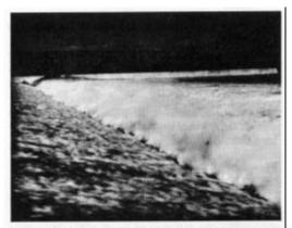
6. Hydraulie jump at the base of a dam.
